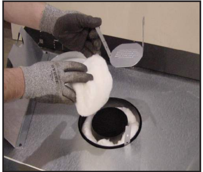
Figure 6.4 (Generic Appliance Shown) Remove the insulation basket and white insulation from the center vent pipe.
