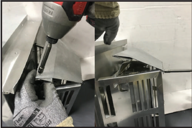
Figure 7.15 Wind Diverter Installed
