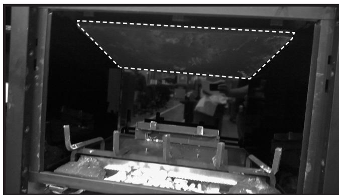
Figure 11.5 Install Top Refractory Panel
