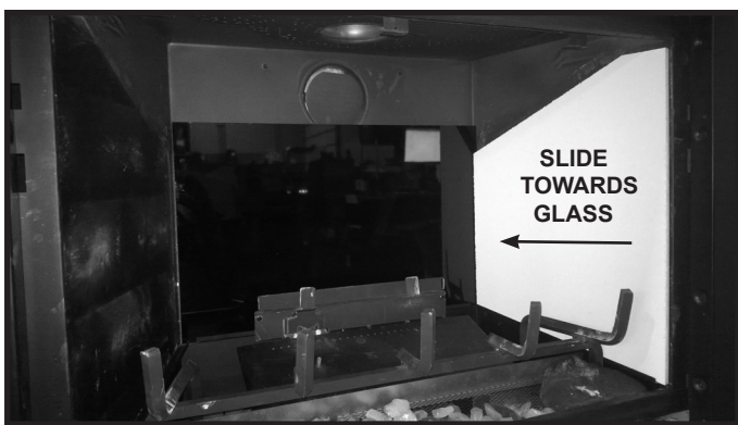
Figure 11.3 Install Rear Glass Panel
