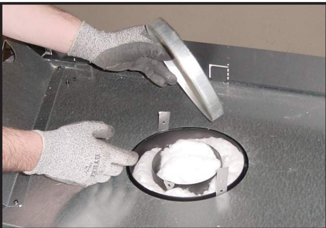
Figure 6.3 (Generic Appliance Shown) Remove the seal cap.
