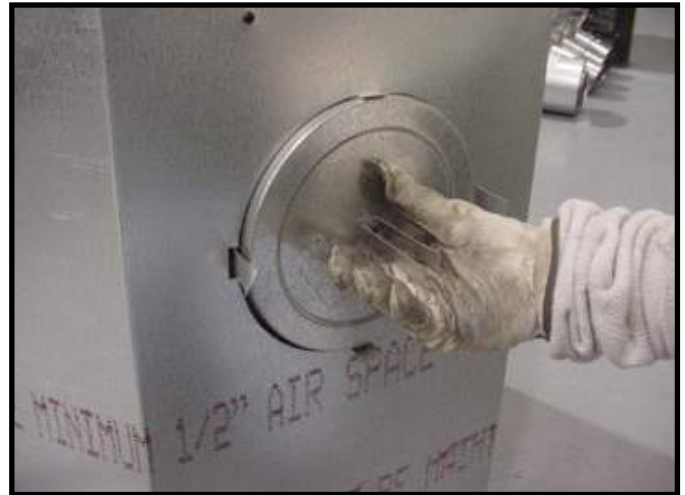
Figure 6.9 (Generic Appliance Shown) Fold the center parts of the retaining band out and use to remove the seal cap.
