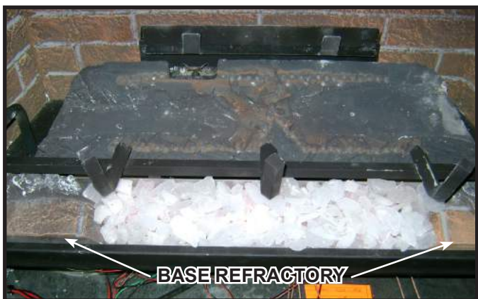
Figure 11.6 Install Base Refractory
