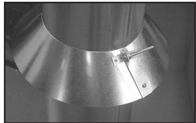
Figure 7.14 insert Bolt into Brackets
